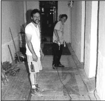
Br. Randy Senecal renovating the basement of the college with Devin Schlosser.
