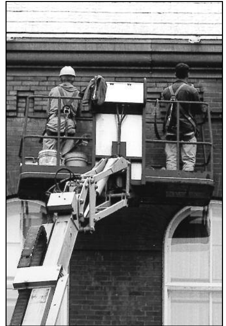
The repairing of the brick work of Michael Hall.
