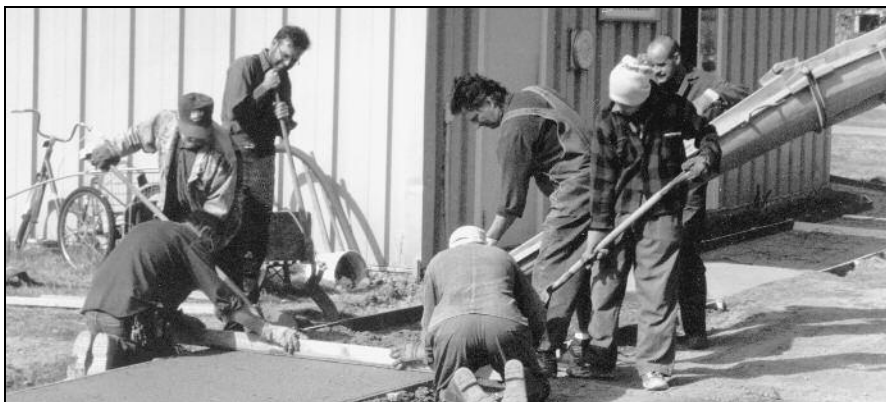
Pouring the sidewalk from the abbey to the car garage.
