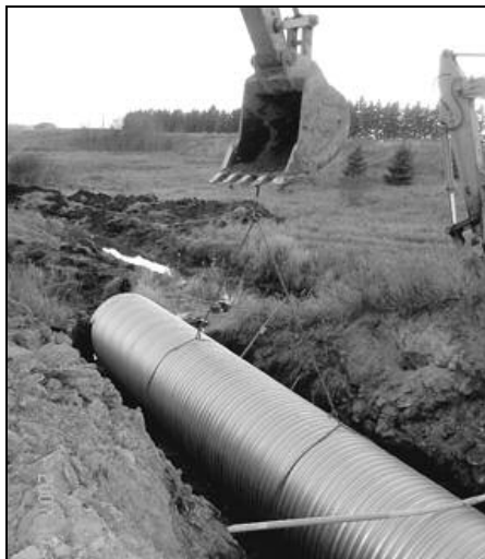
A culvert was installed on the road leading to the abbey.
